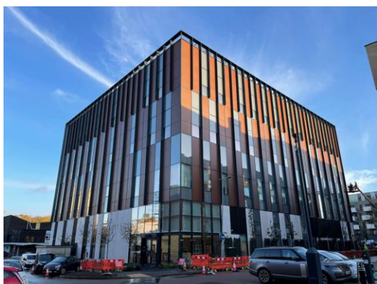
Image: The new Autolus building
